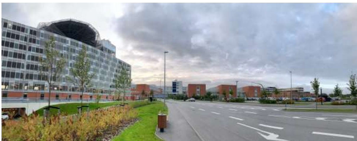
Figure 1 View at main entrance to Orthopaedic Department building
